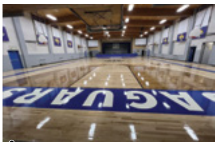
Over the summer, the GSAA gym floor was refinished and repainted.
