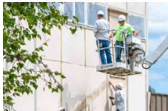
Volunteers spruce up the gymnasium with new paint, windows and siding.
