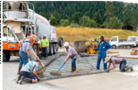
In addition to new lighting and ceiling tiles, volunteers pour new concrete.
