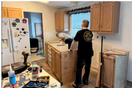
Volunteers reinstall the repaired kitchen cabinets.
