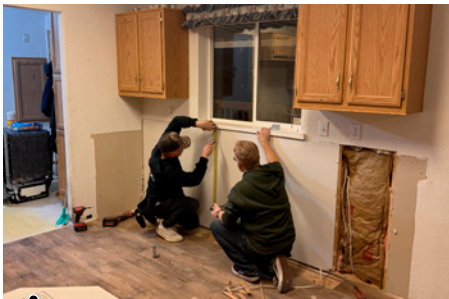
Ian Nesteruk (left) and Jason Lennon (right) repair kitchen drywall.
