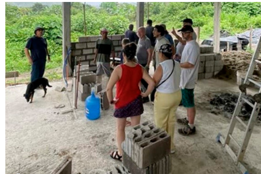
Wasilla Church volunteers help construct a treatment room.
