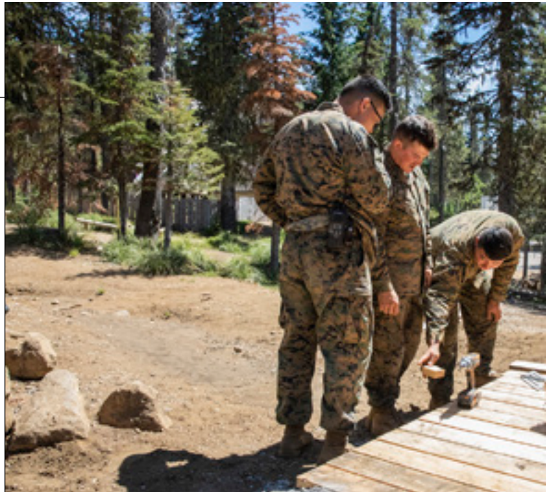
The Marines built new wooden lifeguard towers on the docks, a new blob tower and a new deck for a cabin. They also cut down dead trees, and they rebuilt the retaining wall by the lodge.
