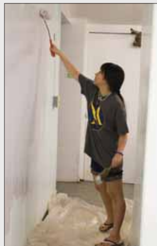
Christine Kim is part of the paint crew during the mission to renovate Hawaii's Kahili Mountain Park.
