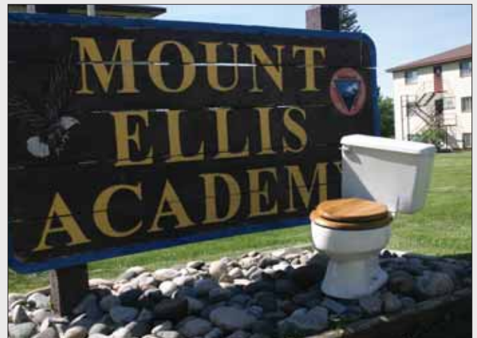
Mount Ellis Academy won a $500,000 grant with the Kohl's Cares competition last year and has been working strategically since that time to upgrade the academy's sewer system.
