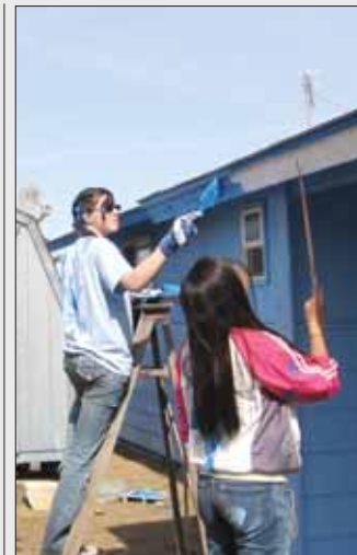
UCA students work on painting a house inside the Yakima Indian Reservation during their recent mission trip.
