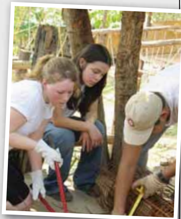
Skagit Academy students work together laying the foundation for a bathroom facility in Bongti, Thailand.
