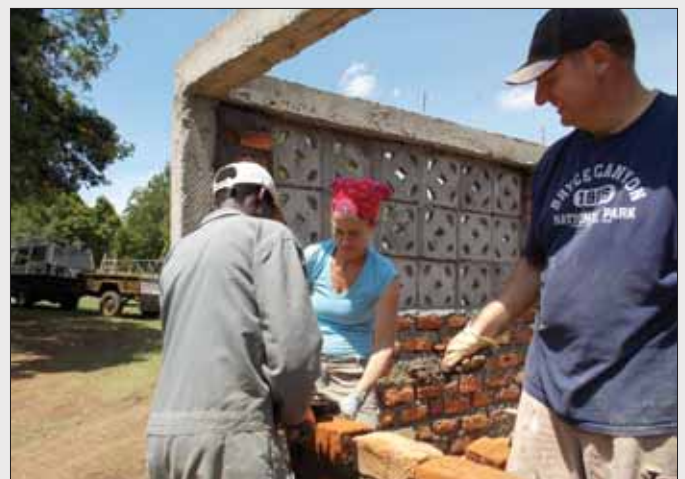
Shelby Vercio and Greg Allen finish the last wall of the project.
